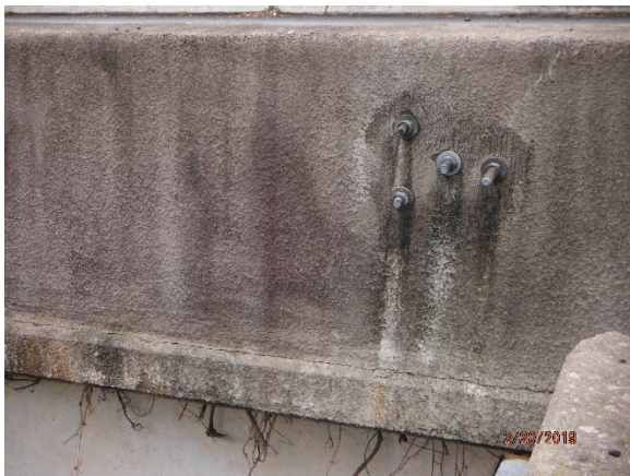
Photo 5. Texture Material on Wall (Spray-Applied)
