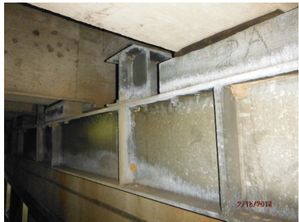
Photo 6. I-Beams to Increase Track Clearance
