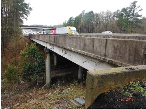
Photo 1. East Side View of Bridge.
