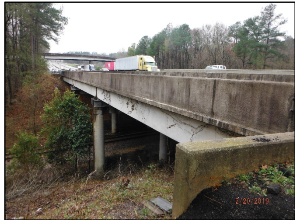
Photo 1 – I-26 Bridge over the CSX Railway in Richland County, SC.
