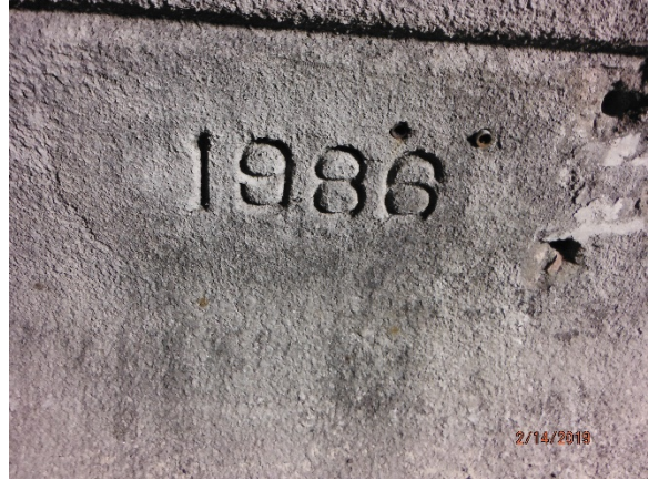
Photo 2. Date Stamp on Bridge
